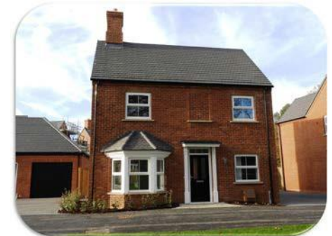
New homes on the former RAF Upwood clinic site, Bury
